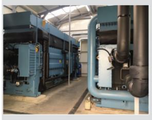
There was an estimation that after the "heat recovery project" at PE, steam generation would be reduced. In order to produce required amount of steam, two new hot water vam chiller machines have been bought to utilize the waste heat of the engines jacket water and Chips Plant column water. A new heat exchanger was installed at Chips Plant to utilize the heat of the vapors of the column to generate hot water to operate new vam chillers.
